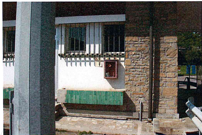
8 Via Braia LAT: 44°36'51,08" LONG: 8°12'45,08" - Esterno
